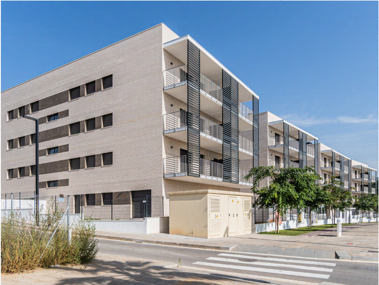
The Edifici Miranada development in Sitges, one of Spain's most expensive rental markets. Thanks to AA energy ratings, communal heat pumps, solar energy systems, and careful orientation, shading, and cross-ventilation, energy costs here are half of the area's average. (Credit: Cohabitac)
